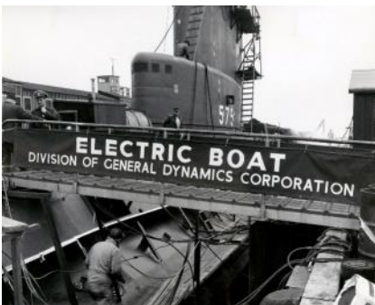
USS Seawolf during fitting-out process after launching. Fitting-out of a nuclear submarine includes installation of the reactor and eventual dockside testing of the power plant ahead of sea trials.
